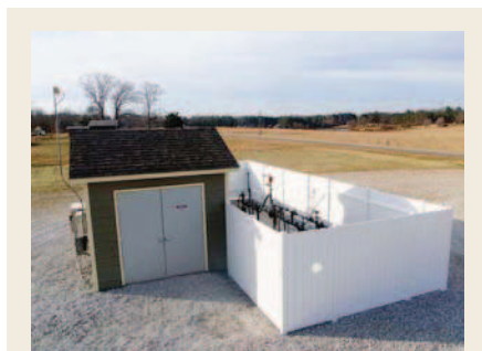
Fig. 4. Housing of the surface unit for Smith Lift's hydraulic diaphragm insertable pump shows the surface unit's small footprint.
